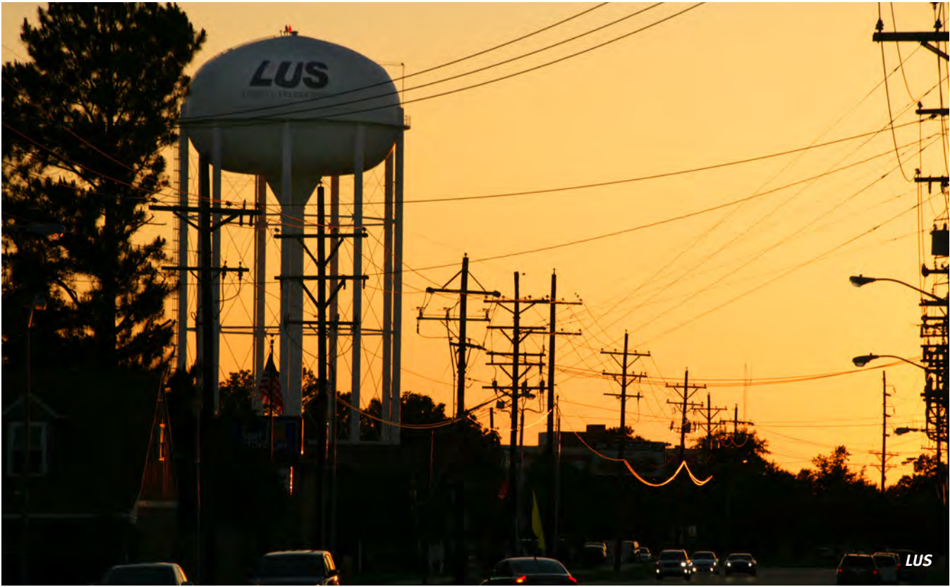
LUS managed water tower and power lines
