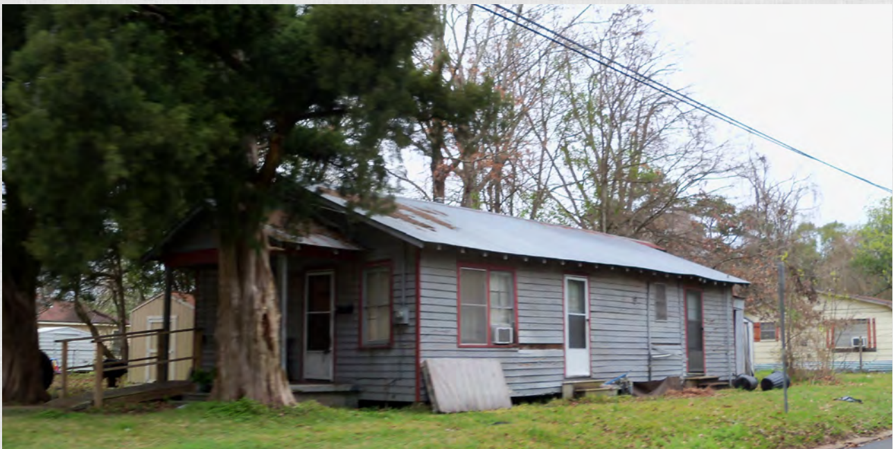
Simcoe Street: Housing in need of repair
